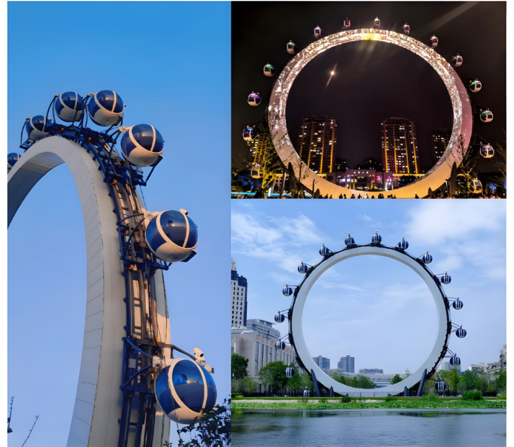
▶ 嘉兴 49米无轴摩天轮—“秀水年华” Jiaxing 49m shaftless Ferris wheel—“Xiushui Nianhua”
